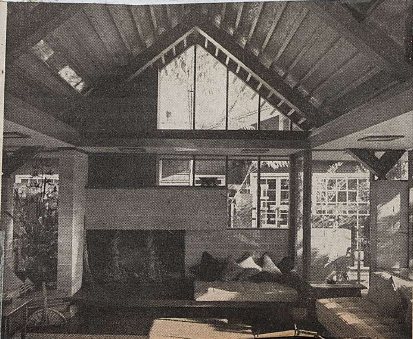
Striking interior of Whifler's home is personified in this view of living room. Note how inobtrusively the concrete block columns reach to meet the pointed steel frames, leaving a wide area for light-admitting glass. Raised hearth and floating lower ceiling accentuate airiness of interior.
