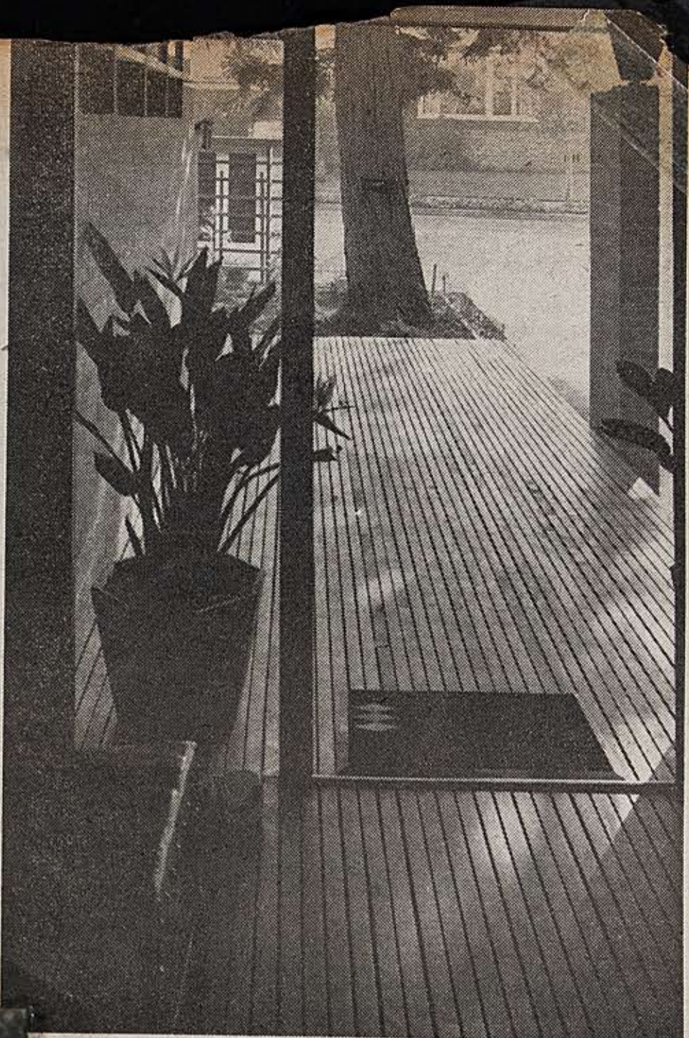
Use of steel frame allows gabled roof and protective overhang to reach far out over entryway with minimal obstructive support, even though it's studded with glass door, wall.
